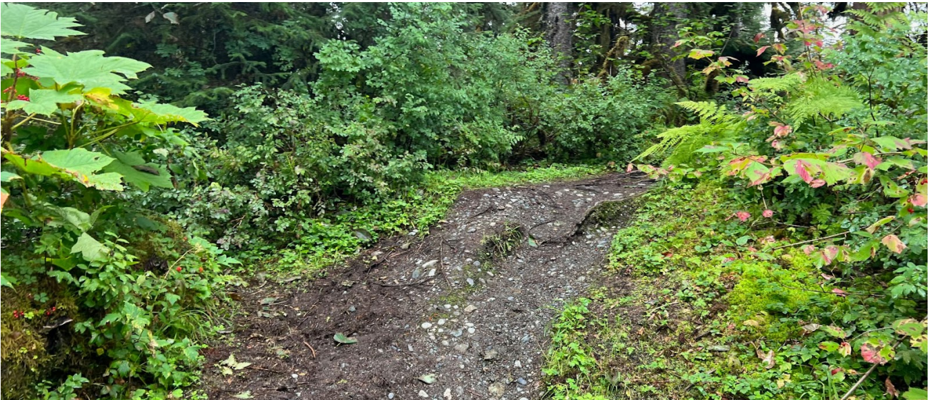
An improved, hardened section of the Situk River Trail; Photo: Haley Johnston
