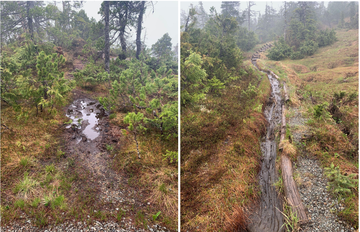
Trail and resource damage along the One Duck Trail; Photos: Haley Johnston
